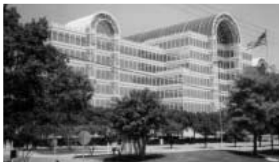
No, this 1.6 million sq. ft. building wasn't our meeting site either. The Infomart in Dallas, just a few blocks from our meeting site, is billed as the world's largest technology community; it houses a mix of technical companies, data centers, telecom switches, fiber optic networks, and offices.
